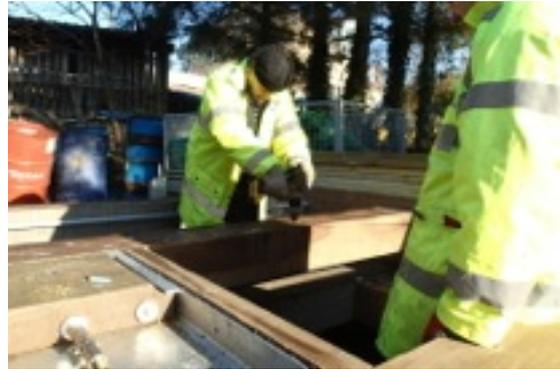
Back on the gate, the planks were removed so that the pilot holes could be drilled out to full depth.
