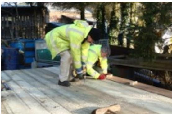
The planks for the gate were already cut, so they were laid out on the gate and the fixing holes drilled through them almost as quick as the positions were marked on the planks.
