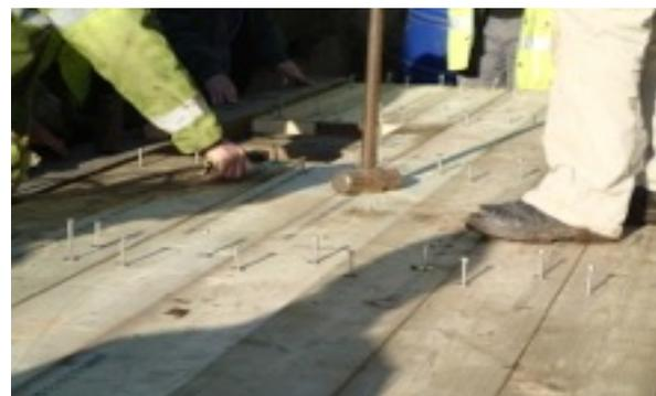
The planks were then finally fitted, tapped down as necessary, and coach screws installed ready for tightening
