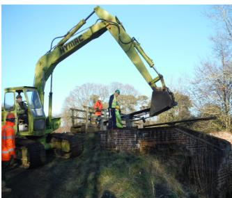
upright posts. The posts were then sawn down to make exact fit to the beam boxes. The balance beams were then lifted and with a lot of juggling and minor adjustments with the grinder fitted to the gates. The angle of the beams had to set at 3.5 degrees. These
