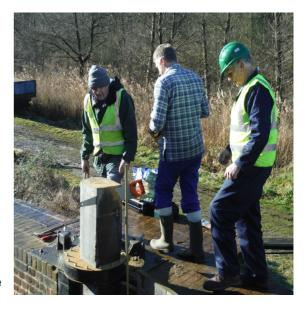
beam, but the path side one is still not clearing the bottom of the lock chamber, so it looks like we will have to lift the gate and inspect and shim up later on. Work finished about 4pm the site was cleared and all tools locked up.
