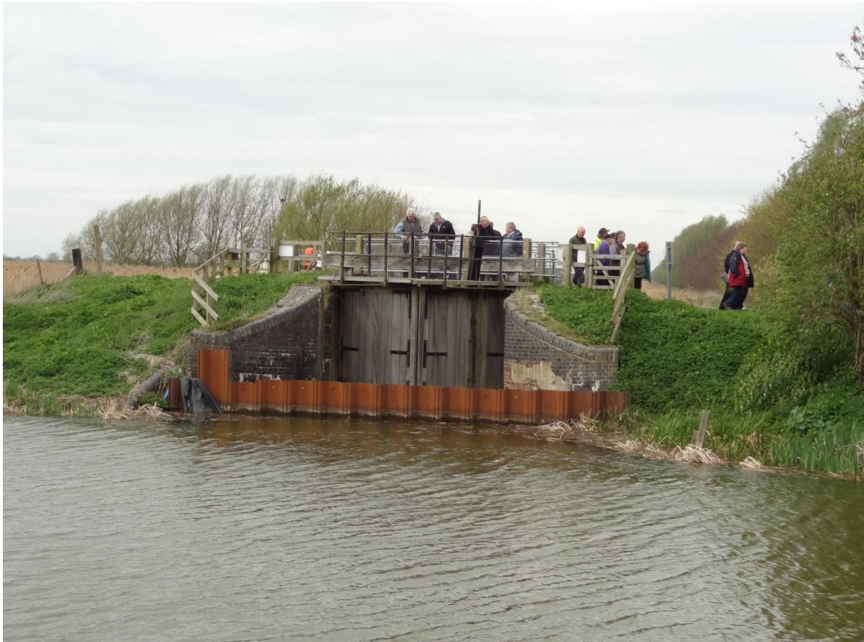
Welches Dam Lock (Photo Ivan Cane – note piling does not reach right hand side)
