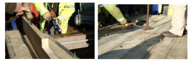
The planks were then finally fitted, tapped down as necessary, and coach screws installed ready for tightening
