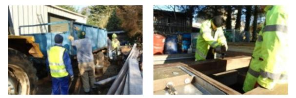
Back on the gate, the planks were removed so that the pilot holes could be drilled out to full depth.
