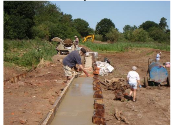
April 2017 Concreting behind the piling
