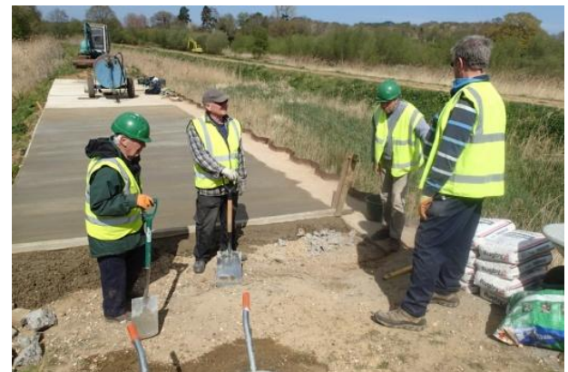
April 2017 Concreting the top slab
