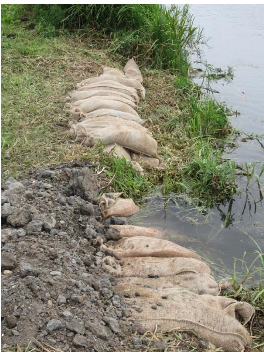
The area for trial was strimmed to ground level and the vegetation removed. Approximately 40 sand bags were filled from the heap of granular material opposite the mill building. The material was mixed with OPC at a ratio of 15:1.
