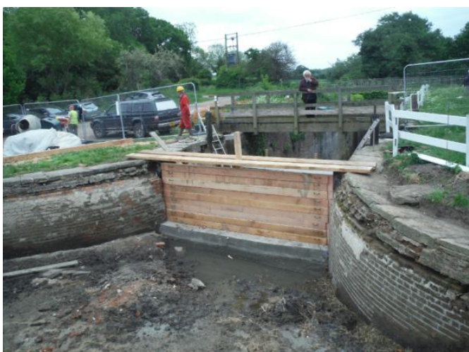
Stop planks in place
