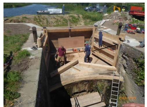
Hargreaves staff installing the gates
