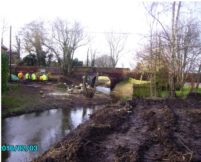
The trees growing in the silt have been removed and the canal has been re-profiled to its original dimensions on the Granary side. Wherries used to be able to turn round in the winding area in front of the bridge. They would be unable to turn here at present, as part of the winding area is now under the car park on the right.
