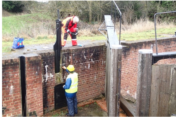
Replacement lock paddle rod being installed (two pictures)
