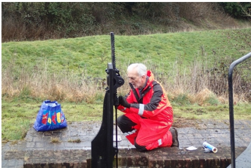
Replacement lock paddle rod being installed (two pictures)
