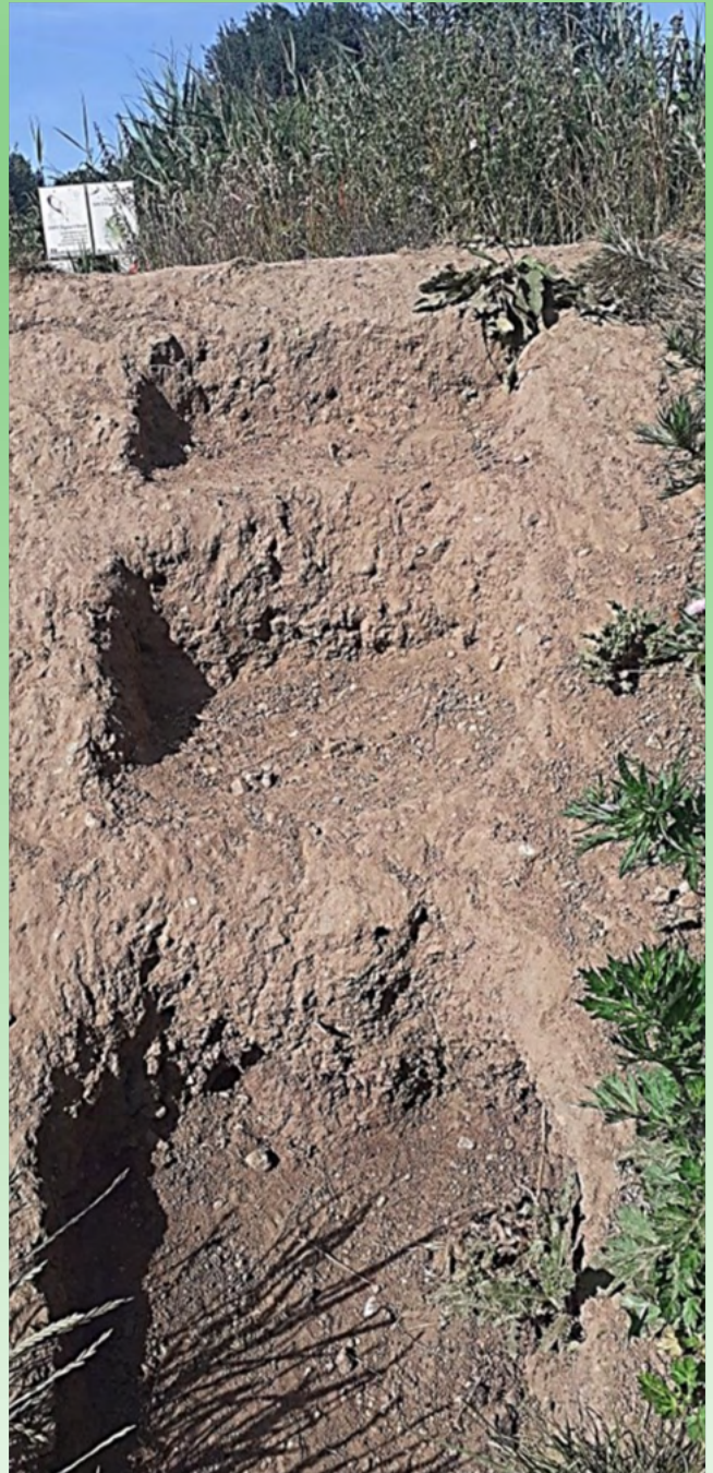
'Steps' cut into canal bank
