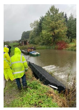
The platform was located with three piles 3.2m long.
