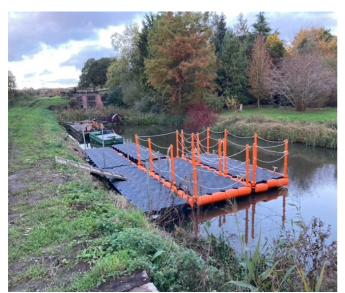
A 5m by 2m pontoon was assembled on the bank complete with hand rails, outboard bracket, fenders, etc
