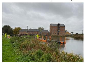
A 5m  $\times$  1.5m platform was assembled, launched and taken to Ebridge mill pond using the small pontoon. An area of the bank was strimmed back. The platform was placed adjacent to the existing one to form a double platform.
